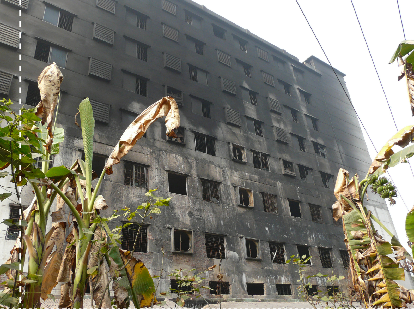
The Tazreen Fashions factory building in Bangladesh where a fire raged in 2012.
